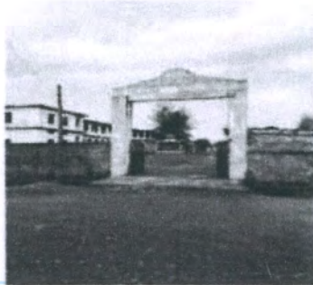
Starting Point ( chainage 00+000 )
