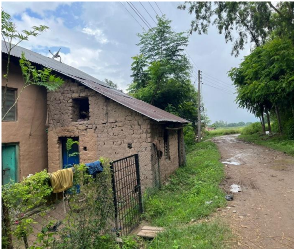
Structure likely to be affected (Ch: 4+260)
