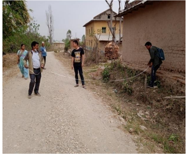
Measuring width of existing road
