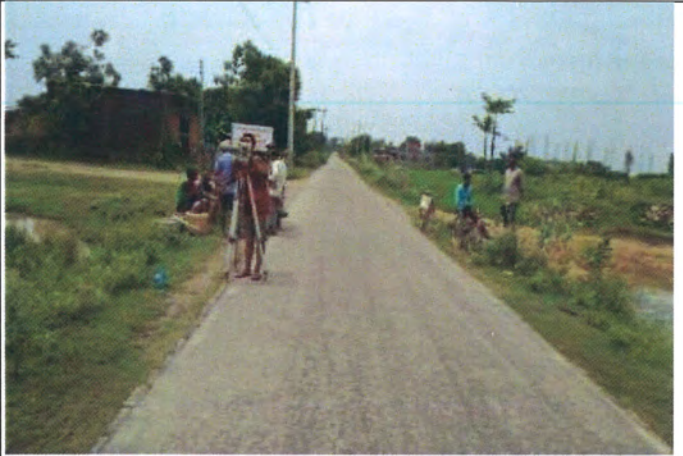
Photograph 10: Road Alignment at Chainage 13+090
