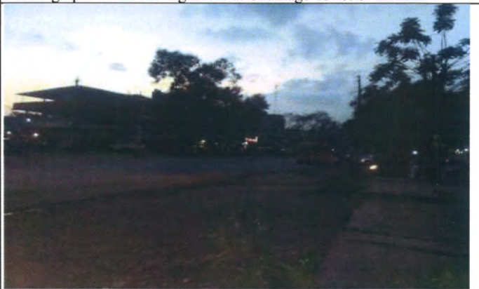
PHOTOGRAPH 12: ENDPOINT KHAIRENI AT MAHENDRA HIGHWAY AT CHAINAGE 22+820
