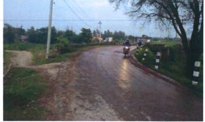
PHOTOGRAPH 8: ROAD SURFACE, DELINEATOR POSTS, SLAB CULVERT AT CHAINAGE 3+400
