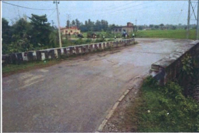
Photograph 9: Slab Culvert at Chainage 3+400
