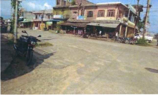
PHOTOGRAPH 7: DHAKDHAIBAZAAR AT CHAINAGE 5+240
